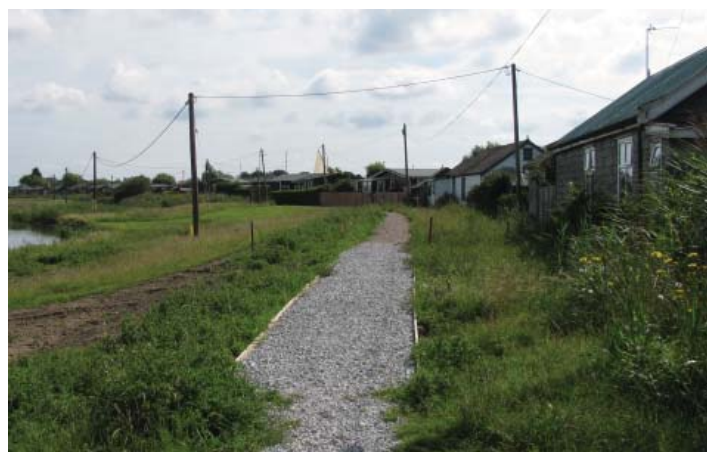
Site of 2007 emergency works
