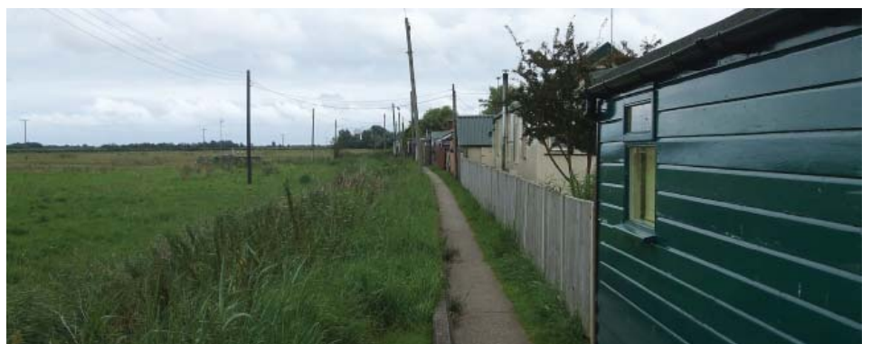
Floodwall behind chalets
