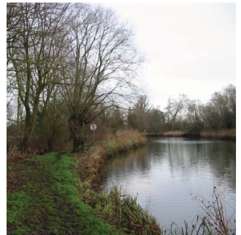
Floodbank along the river downstream of Geldeston Dyke
