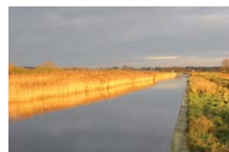
New piling at Short Dyke
