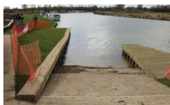
Beccles Yacht Club - new Crest piling and slipway
