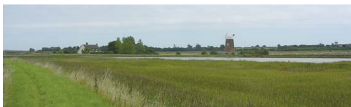
Strengthened flood bank
