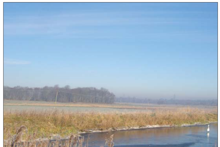
Eroding defences on the River Waveney
