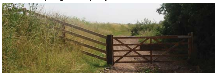
New access fencing for landowner
