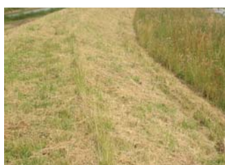
New flood bank
