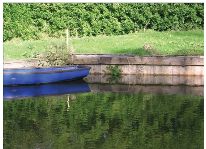
Existing erosion protection (timber piling), River Waveney
