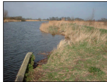
Scour pockets and narrowing road
