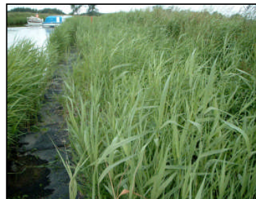
Six months after installation
