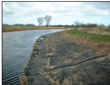
Asphalt matting with reed rhizomes installed underneath to help reed re-growth.
