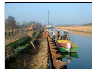
Closure of Short Dyke for re-piling
