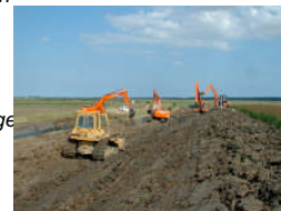
Plant working on new bank at Reedham (Compartment 14)
