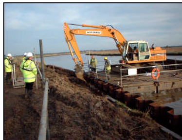
Backfilling to piling, Seven Mile House, River Yare
