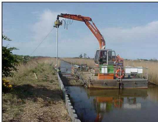
Steel piling installation, Waxham New Cut
