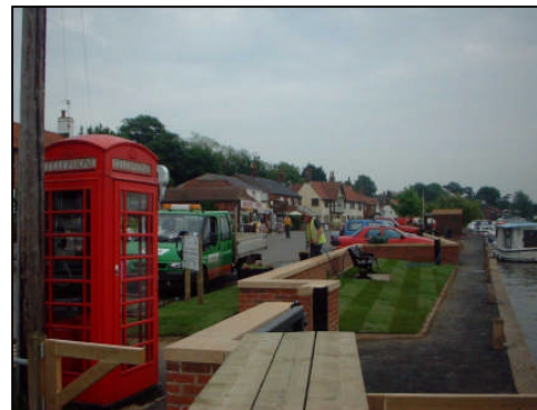
Provision of first time flood defences at Reedham
