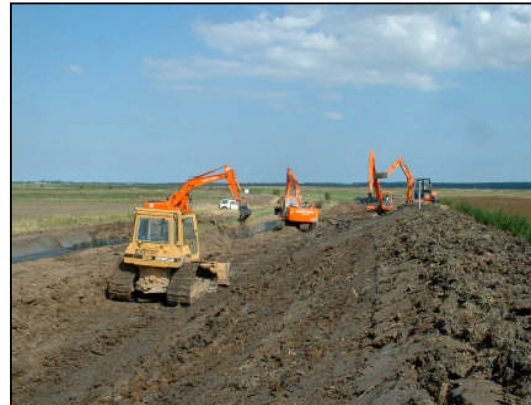
Floodbank strengthening, Reedham Marshes, River Yare
