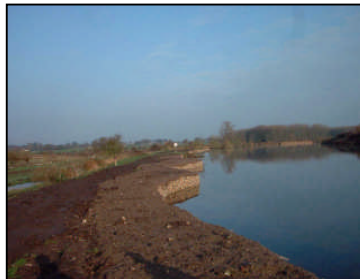
Gabion basket installation
