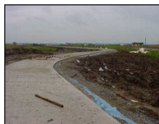
New concrete road, Haddiscoe Island
