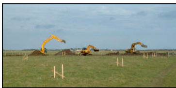
Early stages of set back bank with line and slope profiles visible in foreground
