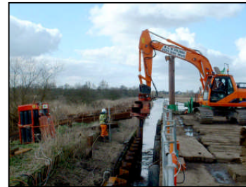
Excavator-mounted vibrating hammer installing piles from river
