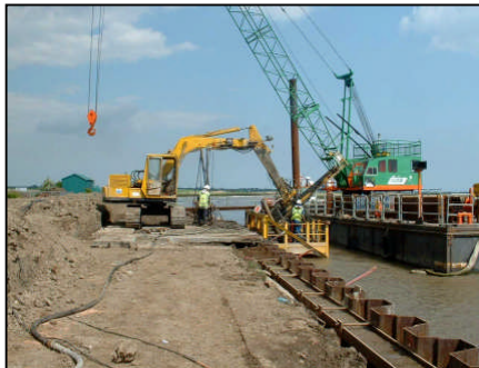
Installing ground anchors
