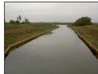
Timber post erosion protection
