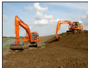
Topsoiling profiled bank
