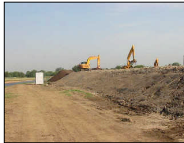
Construction of setback floodbank
