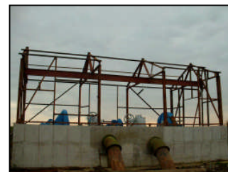
Restoration of historical pump station, Seven Mile House (River Yare)
