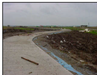
New concrete road, Haddiscoe Island
