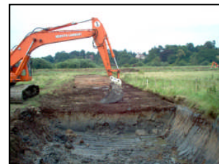
Excavating new soke dyke
