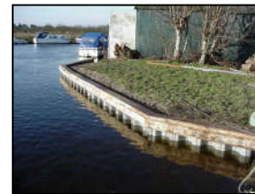
Completed piles in a boatyard
