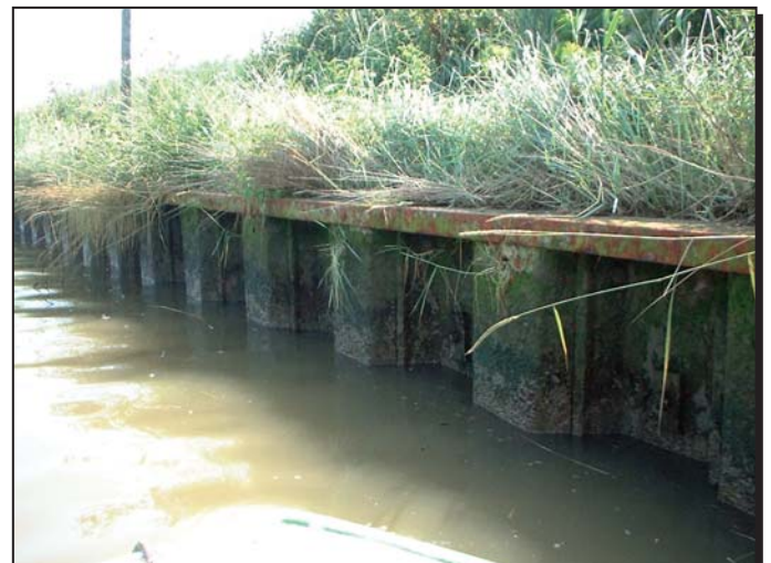
Existing piling along the Cut (railway side).
