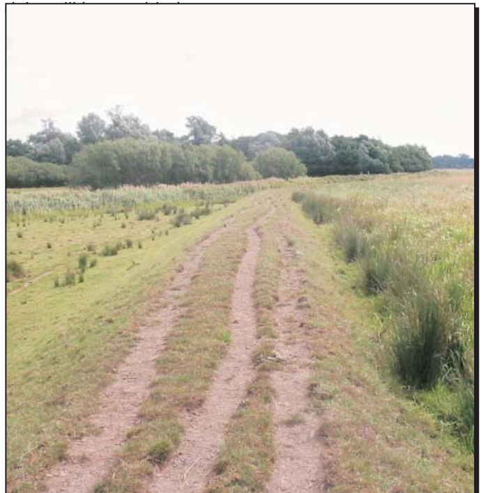
Existing floodbank and rond, Somerleyton Marshes
