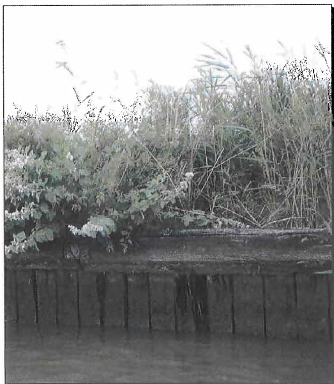
Timber piling - River Chet
