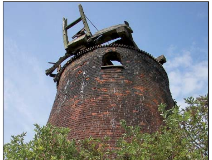
Limpenhoe Drainage Mill
